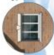
Respectful Windows On exterior windows use 1/2" profile
