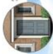
Front Door Panels Use wood frame surrounding door
